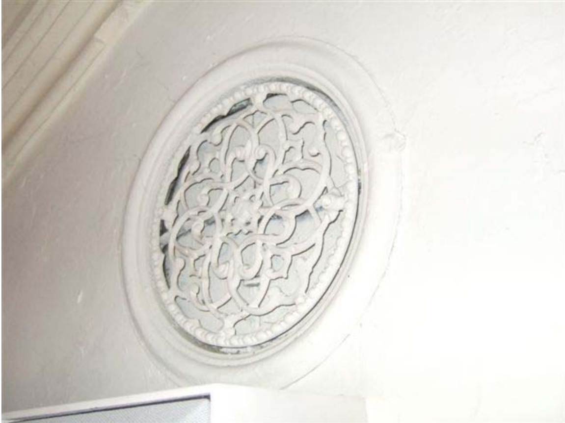
13. Ventilator in gallery.
