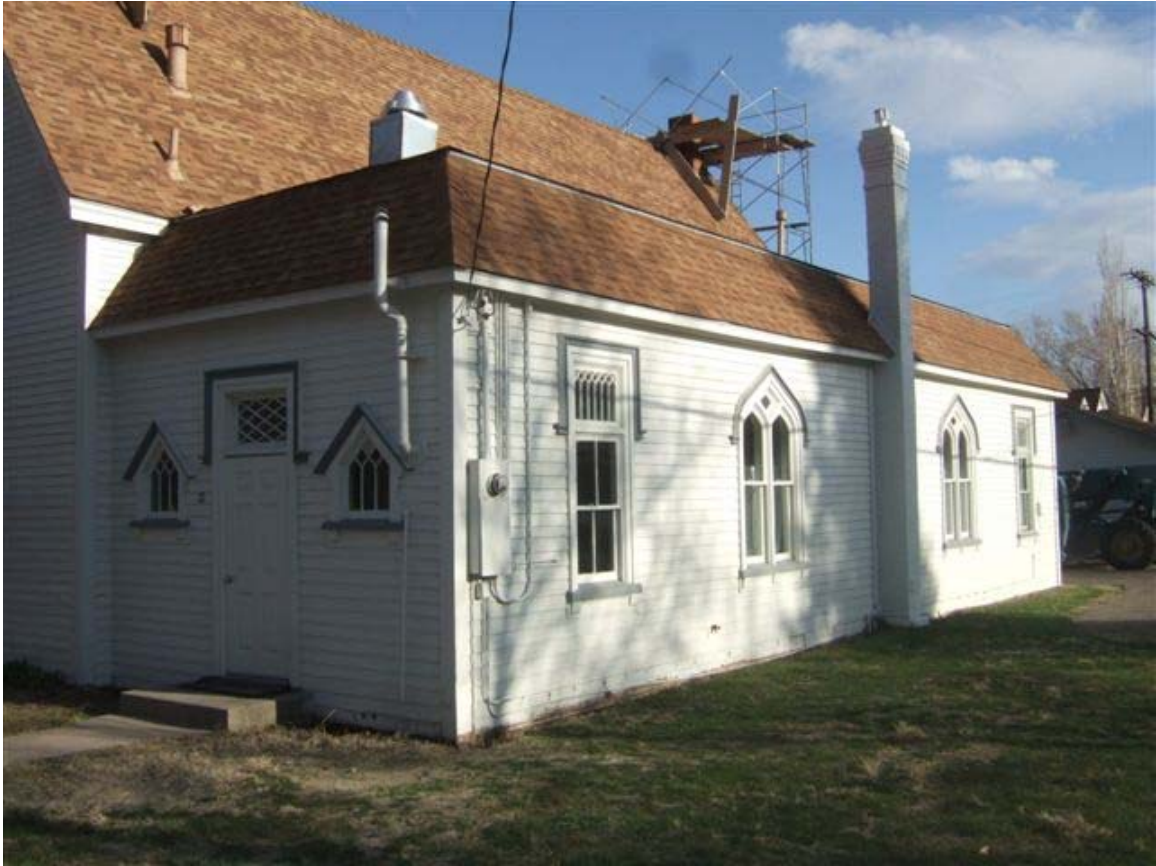
15. North and west sides of 1911 addition.
