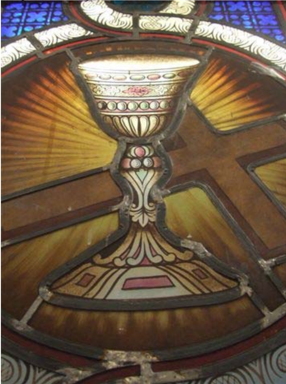
22. Sacristy window detail.
