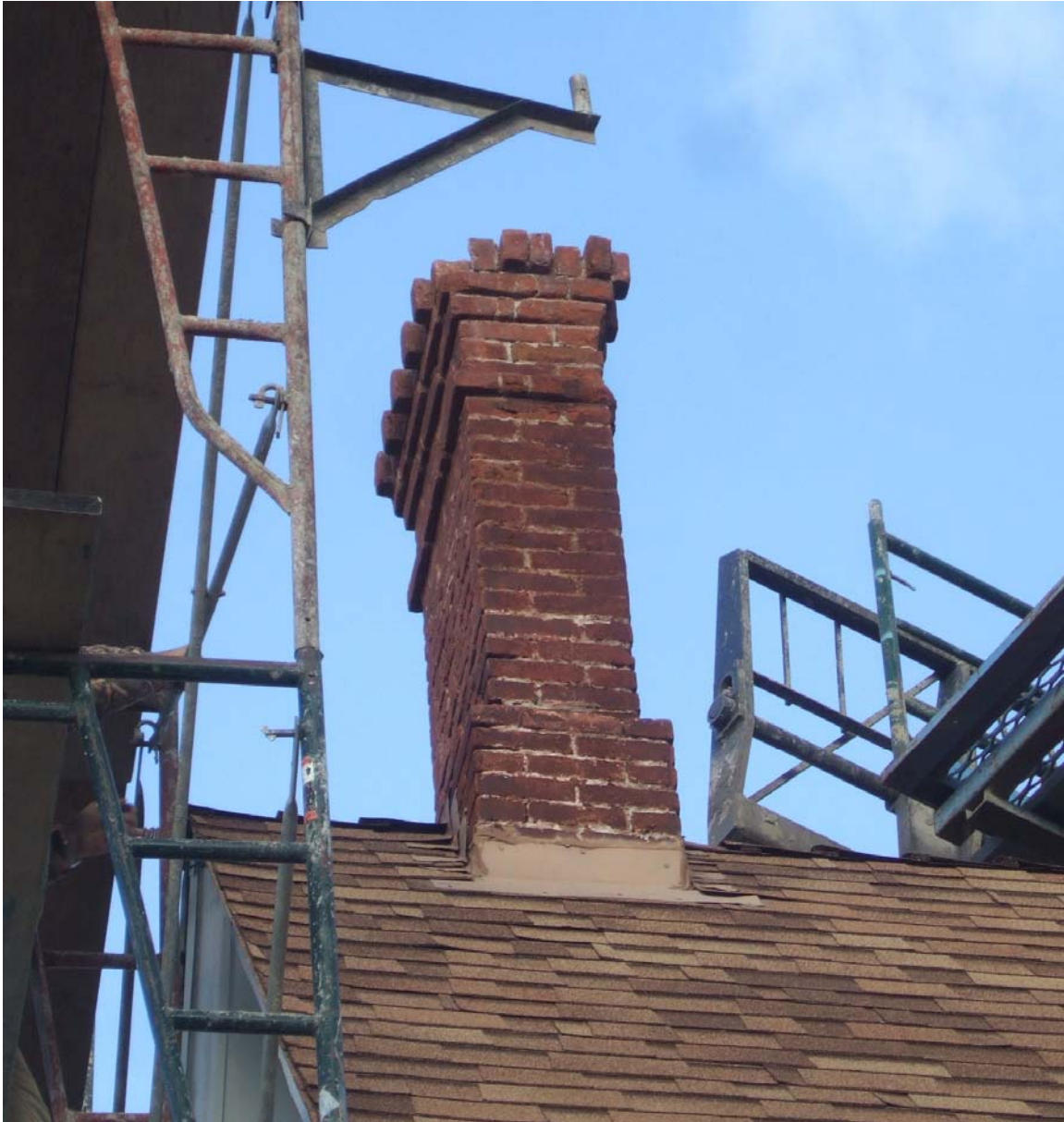
18. One of the 1873-74 flues under repair in March 2008.
