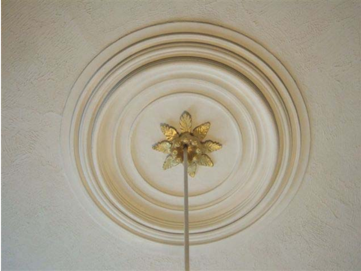
7. Parish hall ceiling medallion.
