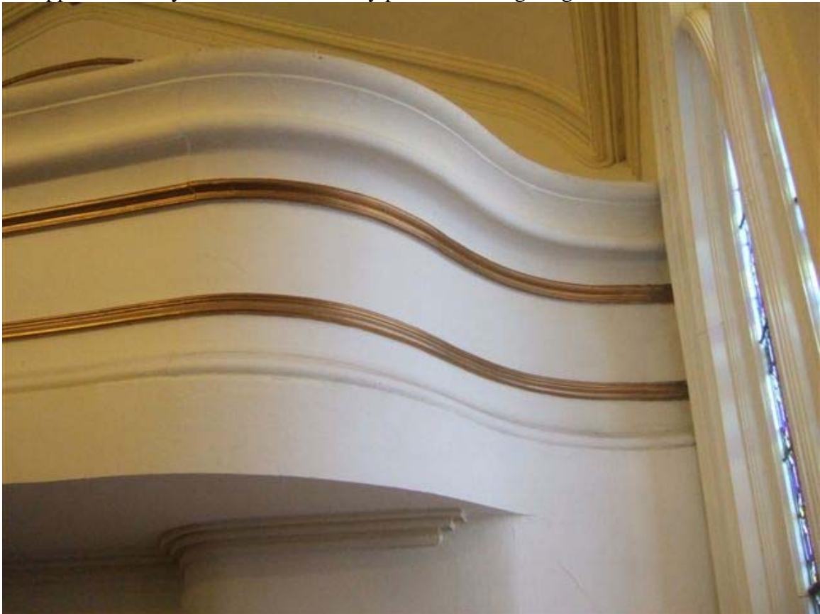
23. Gallery railing detail.
